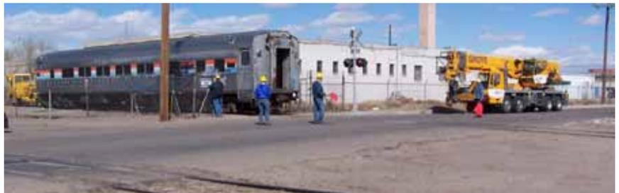
Car mover shifts chair car out of gate and across 8th St to allow a mobile crane from Crane Services access to site for some heavy lifting.
