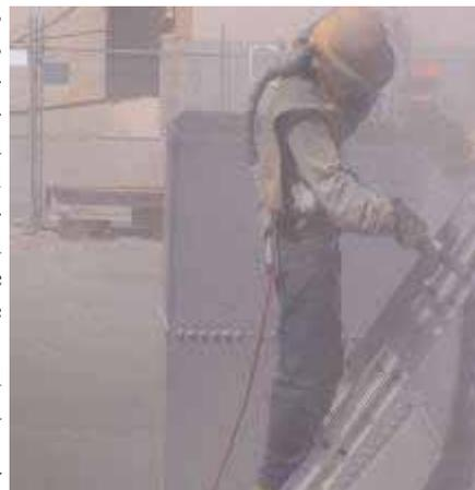
*Above: Working inside the tender's fuel bunker pocket, an R&R employee blasts paint and rust with compressed air and copper slag grit.*
