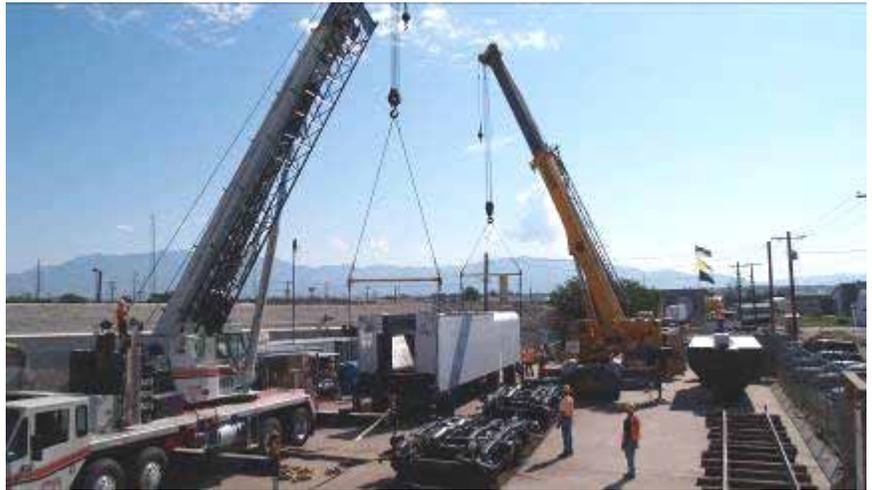
*Against a Sandia Mountain backdrop, the two cranes operate in unison to lift the huge tender body. It floats slowly from the cribbing where it was restored to its freshly restored trucks already back on tracks at bottom center of the photo.*
