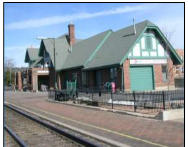
Flagstaff AZ Depot: Designed and built by AT&SF Railway in 1926, this classic Tudor Revival building is now restored, and serves two functions—Amtrak station and Flagstaff's Visitor Center while serving as an icon of the city's rail heritage.
