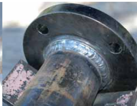
Examples of Rick Kirby's welding prowess. On the left is the junction of the side pipes and the vertical standpipe. On the right is a flange at a check valve.
