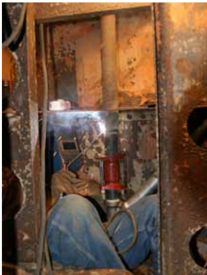
Deep inside the tender, Rick welds while lying on his back in a cramped corner.
