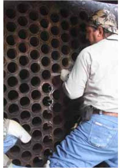
Cutting old flues loose at flue sheet.
