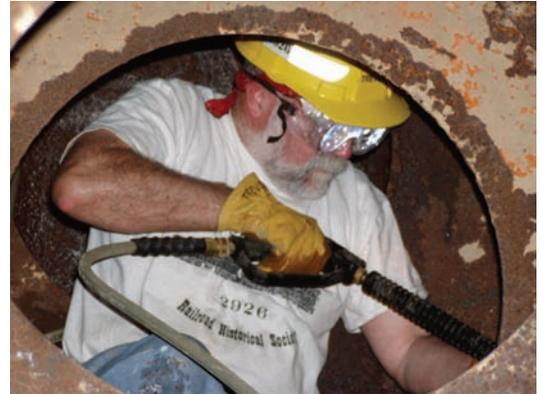
Working in the 2926 tender is much like spelunking. Instead of tight passages and big rocks, tender diving means scrambling through holes in the many baffles that prevent sloshing and add strength. Here, George Trevor attacks the scale.
