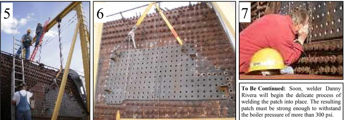
**To Be Continued:** Soon, welder Danny Rivera will begin the delicate process of welding the patch into place. The resulting patch must be strong enough to withstand the boiler pressure of more than 300 psi.
